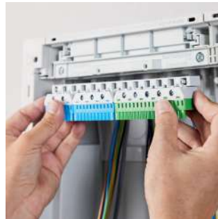
11 The terminal rails with the N/PE Quick-terminals are simply clicked into place from the front; in addition, the cables can also be fixed to the cable support/strain relief fastening
