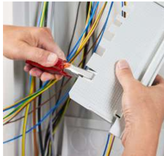
10 Easily break out the knockouts in the slider for cable entry
